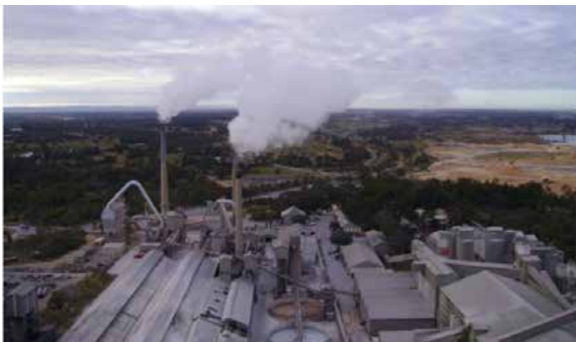
Figure 16. Cockburn Cement Western Australia.
