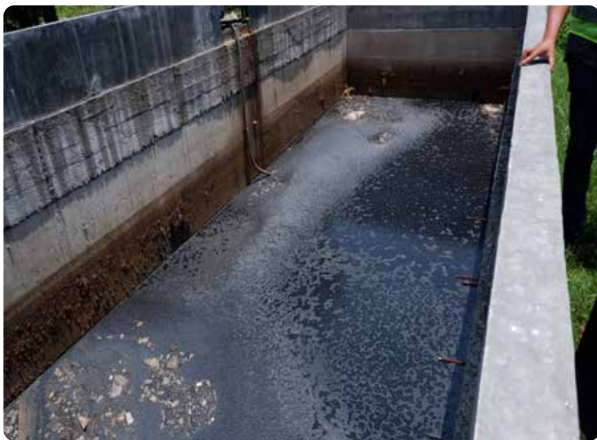
Figure 21. The tank to hold water produced from the Biodrying process without chemicals or biological process. Photo: WALHI
