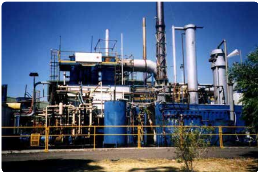
Figure 8. GPCR operating in 24 hour, 7 day cycle for high strength PCB oil/waste. Kwinana Australia 1999. Source: D. Hallett
