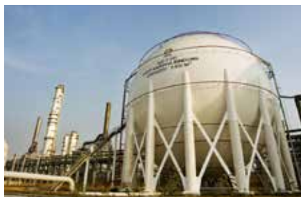
Figure 11. PT TPPI's light naphtha storage tank capacity of 11,400 m 3 . Photo: PT TPPI
