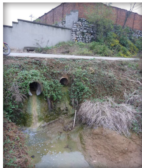
Waste pipe from Dasheng chemical in Zhongxiang dumps water with high arsenic levels. Photo credit: Xie Xinyuan
