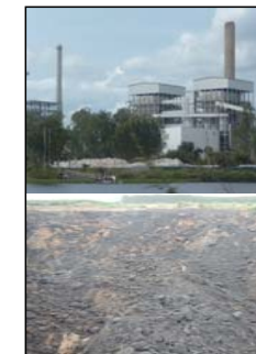
In Tha Tum rural municipality, Prachinburi, Thailand, coal-fired power plants consume at least 700,000 tons of coal every year, supplying electricity and steam power to one of the largest pulp and paper production plants in the country. They also supply energy to over 130 other factories within the 304 Industrial Complex. Mercury releases occur through power plant air emissions and from fly ash disposal. Residents claim coal fly ash is added to the soil on surrounding eucalyptus plantations. Company representatives claim fly ash used to improve the soil on eucalyptus fields only comes from biomass burned at the power plant. Source and photo credit: EARTH
