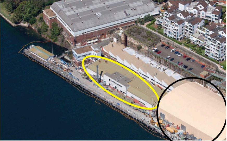
Picture 7. Remediation with odor control enclosure and treatment train. Source: Australian Federal Government (2013)
