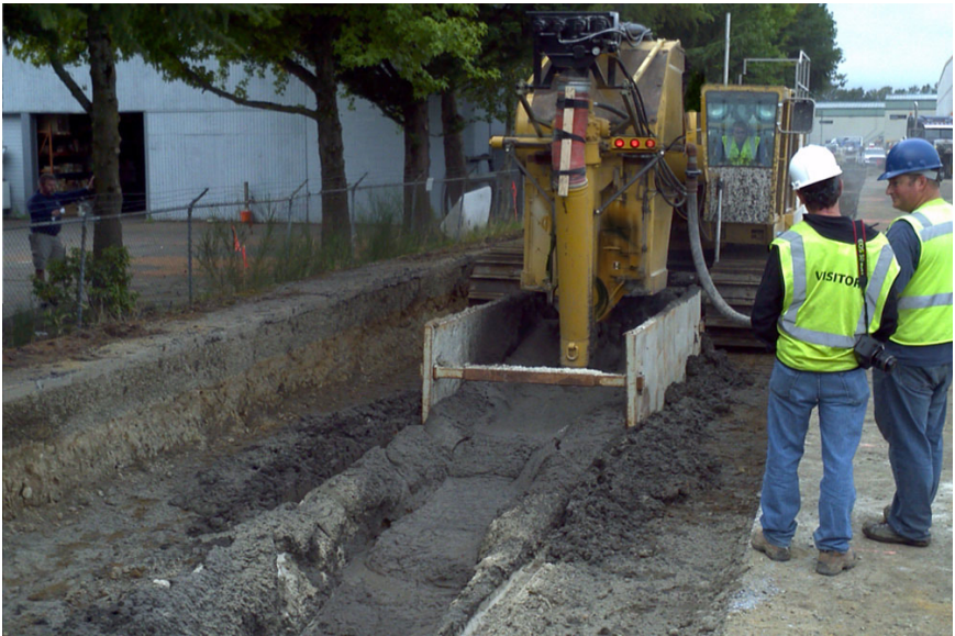
Picture 10. Combined trenching and slurry insertion.
