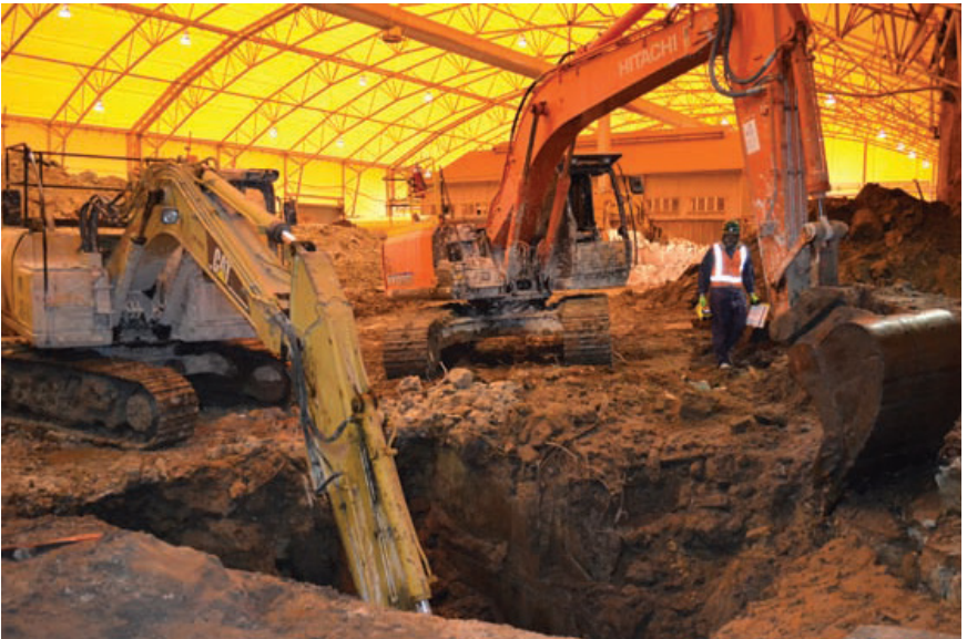
Picture 8. Interior of odor control enclosure during excavation. Source: Australian Federal Government (2013)
