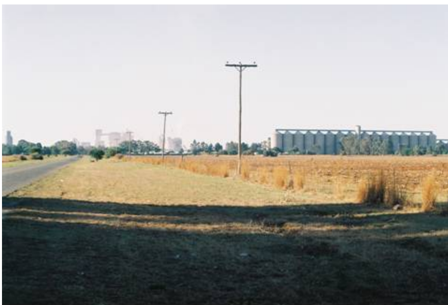
Figure C: Grain storage facilities located next to Holcim cement in Lichtenburg
