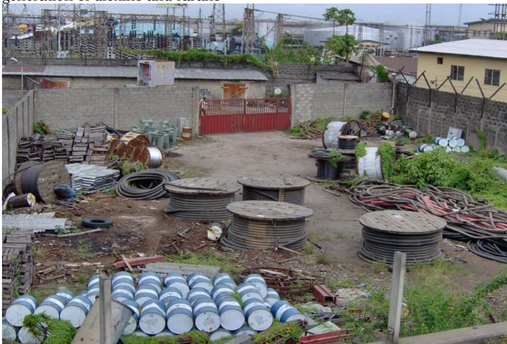
Plate 2: PHCN Workshop with obsolete transformers containing PCBs
