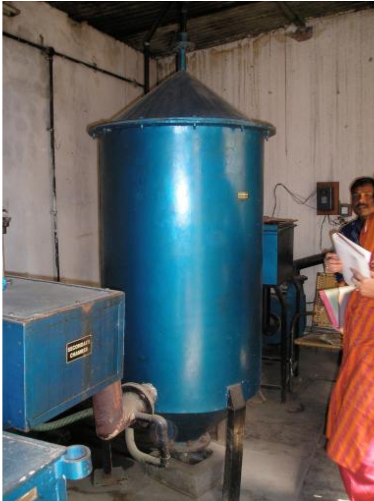
Picture 5: Second chamber of the Queen Mary's Hospital, Lucknow medical waste incinerator Photo by: Upasana Choudhry.
