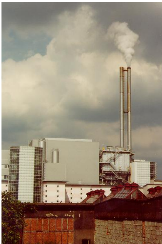
Photo No. 14: Liberec Municipal Waste Incinerator.
