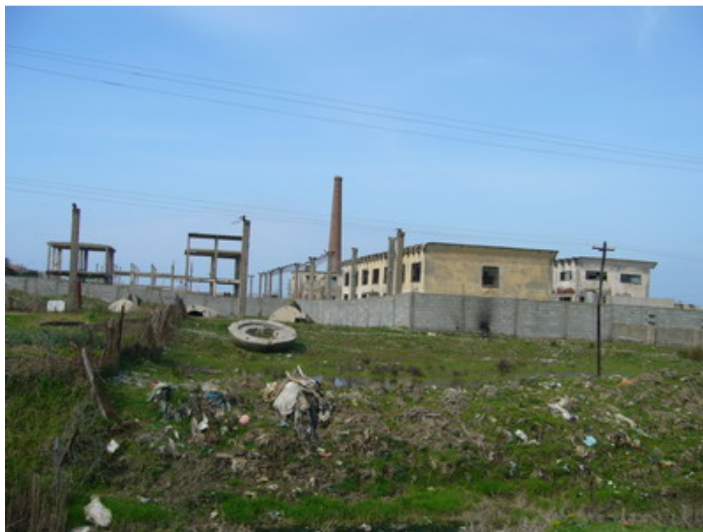
Picture 1: View on the fenced area of the former chemical plant
