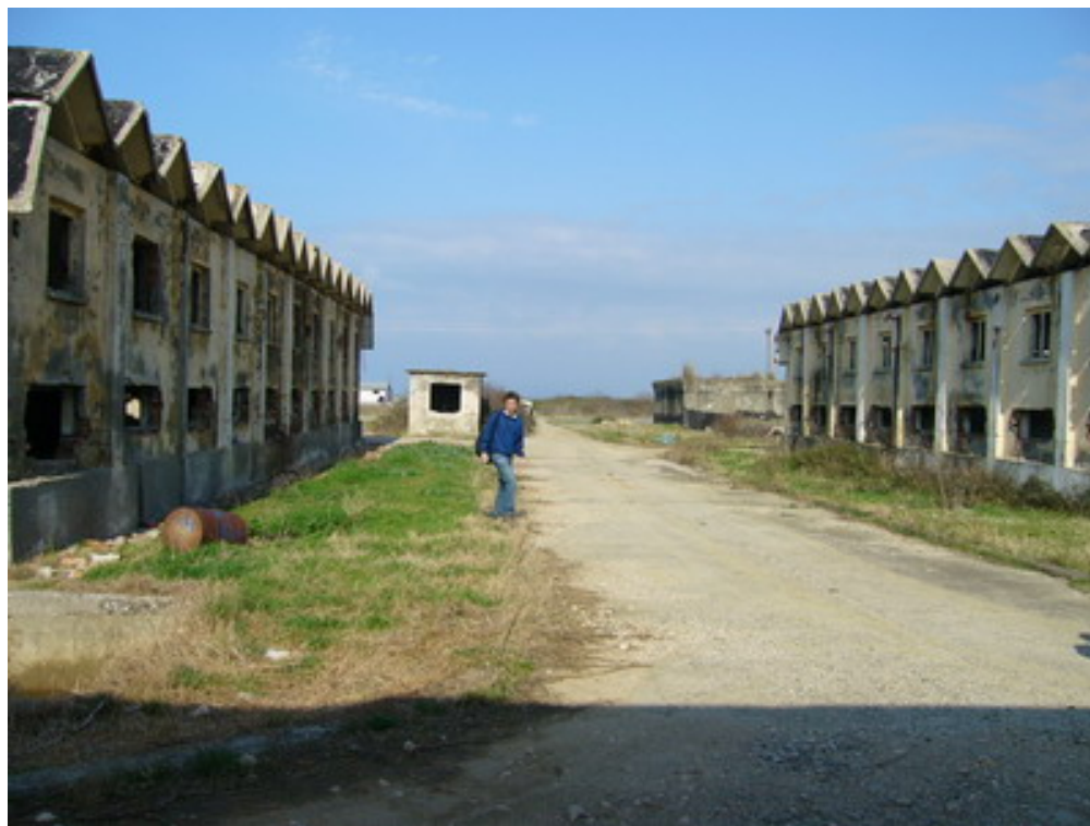
Picture 5: Unsecured storage houses for the obsolete chemical at Bishti Palles.
