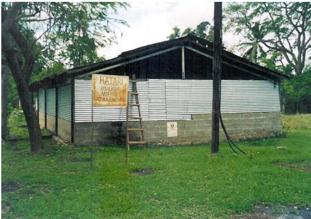
Fig. 5 The new storage facility at Old Korogwe
