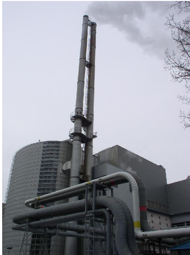
Photo No. 8: MWI Termizo Liberec, January 2005.
