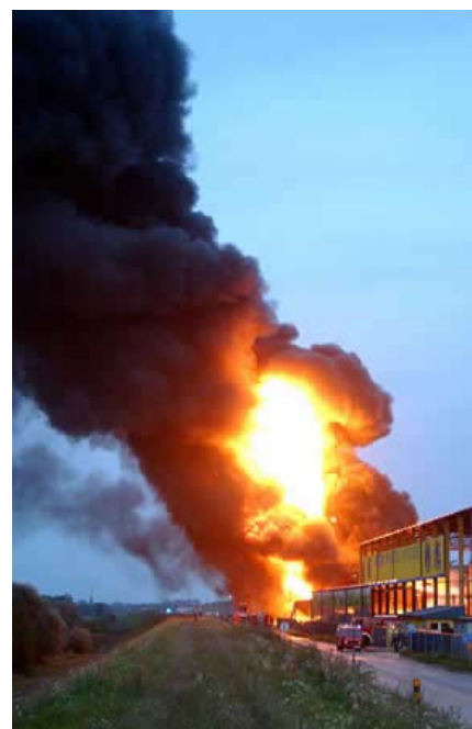
Figure 2: Fire in PUTO incinerator 1
