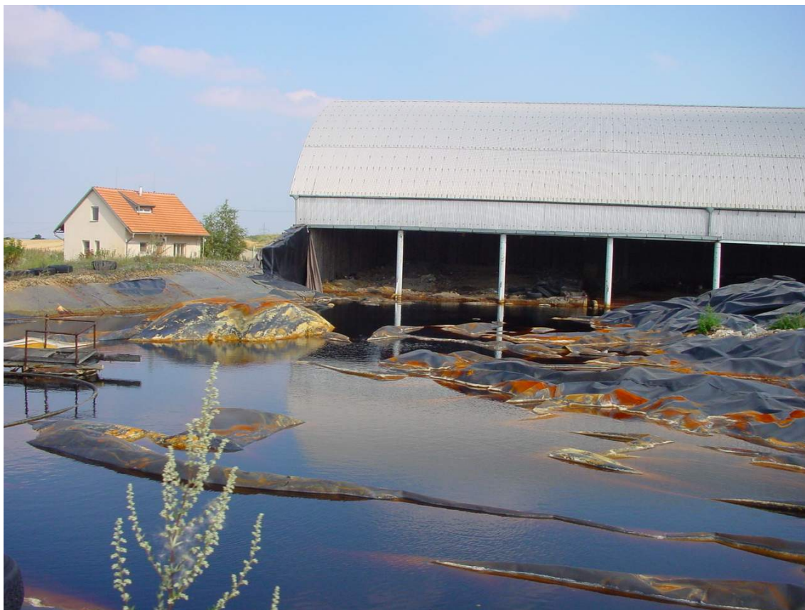
Figure 2: Broken down hazardous waste landfill in Pozdatky
