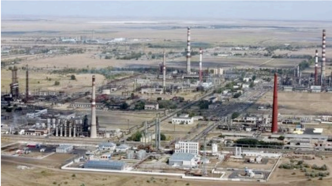
Pavlodar Petrochemical cluster Source: Tengrinews
