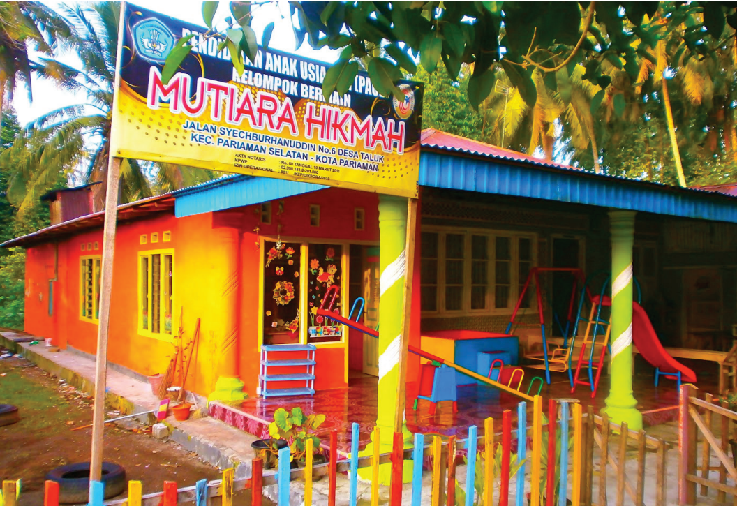
This brightly colored day care center in Indonesia very probably was covered with paints containing high levels of lead.
