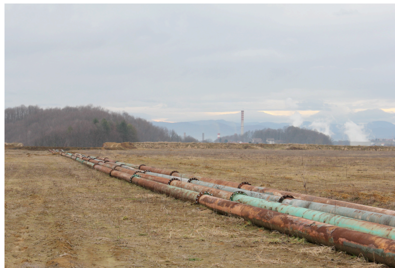
An ash landfill near Tuzla power plant.
